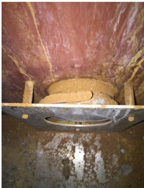
IMG_6019.jpg Before repair
