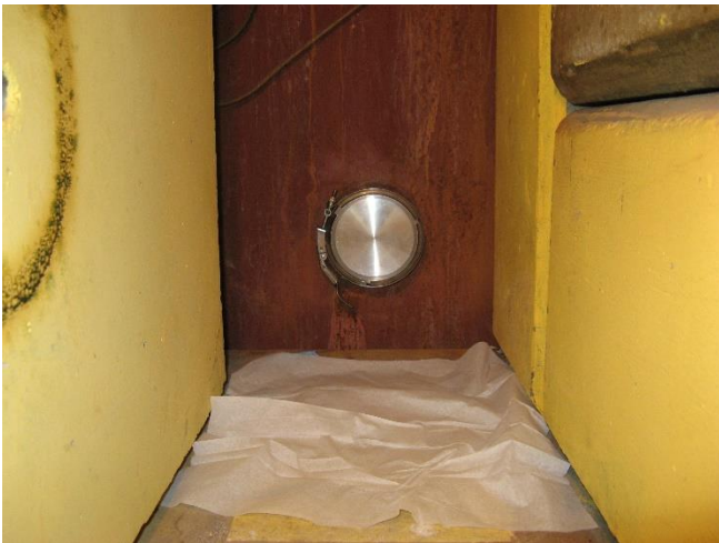
IMG_0449.jpg New Blank-off flange installed
