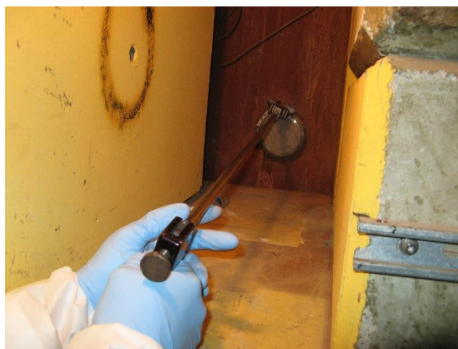
IMG_0434.jpg Removing leaking Blank-off flange
