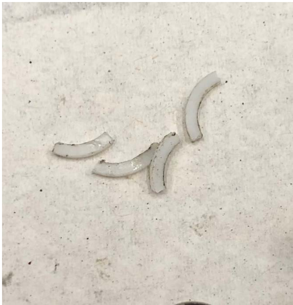
Figure 3: Broken (upon disassembly) PTFE Backup Ring. The material properties have changed to make the PTFE material brittle and possibly worn.
