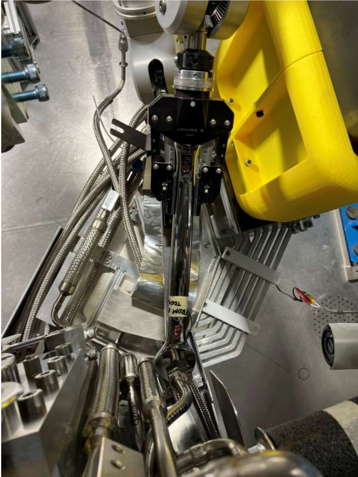
Some interference possible between full size wrench and male side of VCR joint on second to bottom water line.
