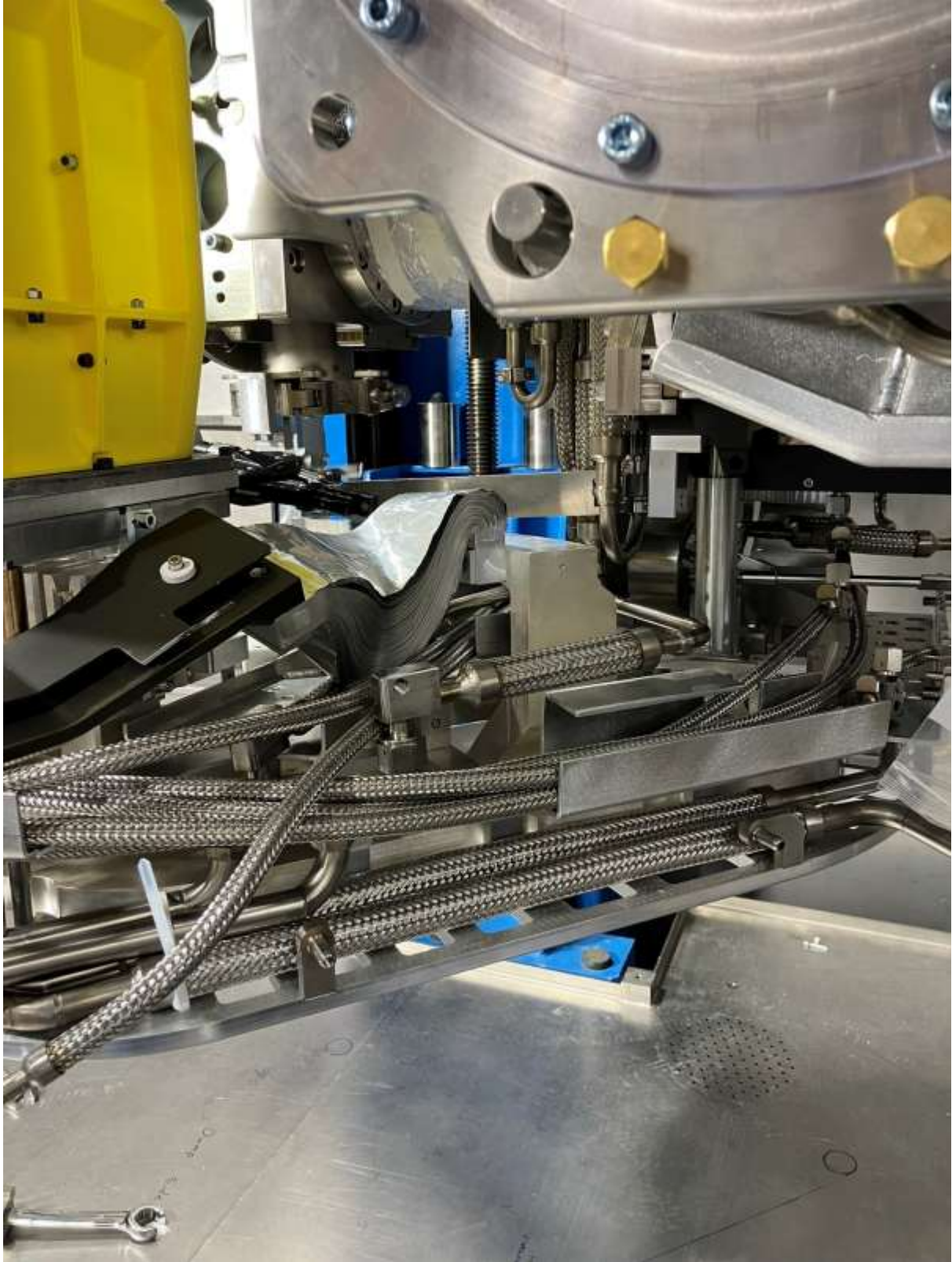
Reach of existing sheet metal barely enough to reach top most water line's VCR joint.
