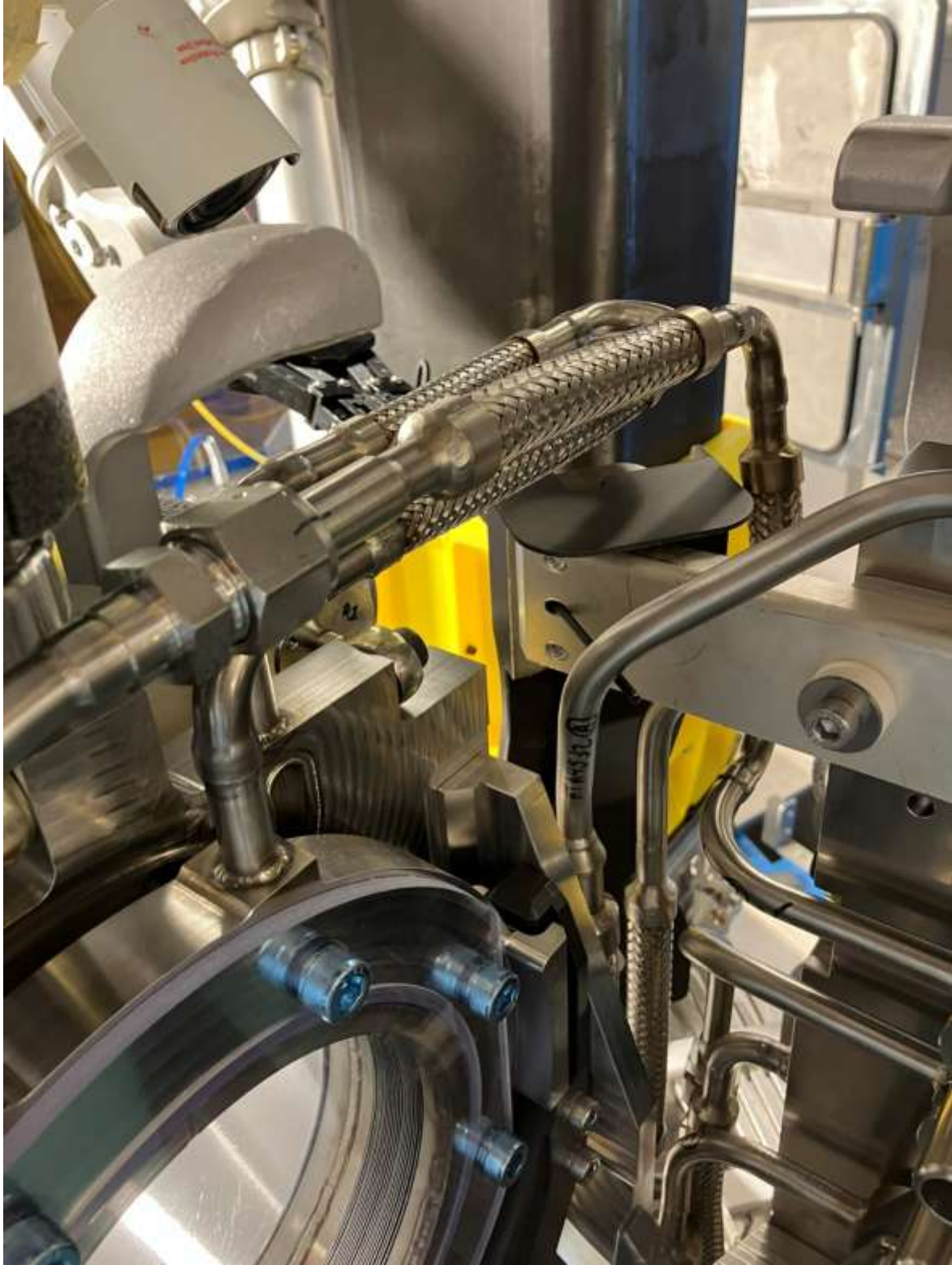
'Pinning' a screw hole on busbar.
