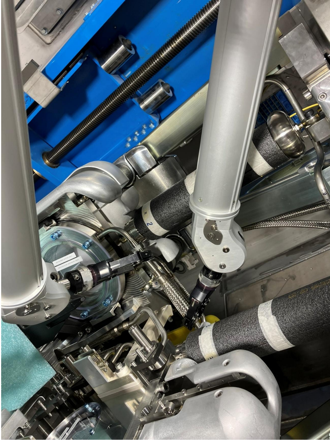
Starting VCR joint on second to top line with difficulty
